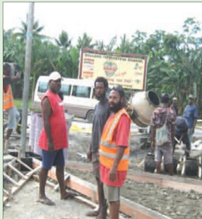
WOKIM NAU: Projek Menesa, Stanley Gaan bilong Better Roads Construction, wantaim tupela wokman bilong em i sanap long nupela raun-about long Madang. Poto: James Kila
